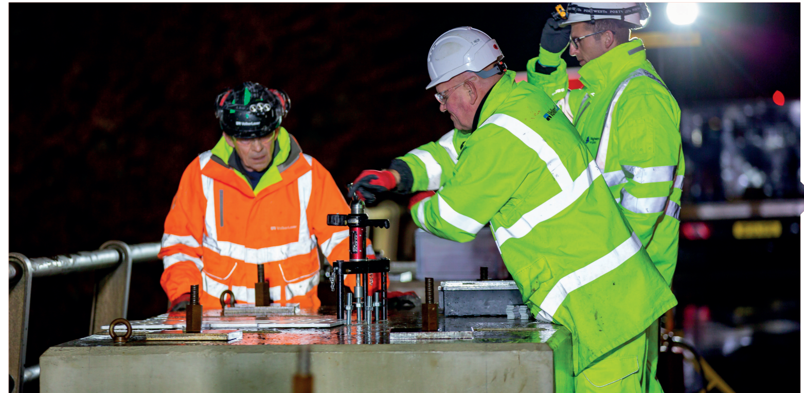
FAST BEAM INSTALLATION ON M1 JUNCTIONS 21A - 23A.
