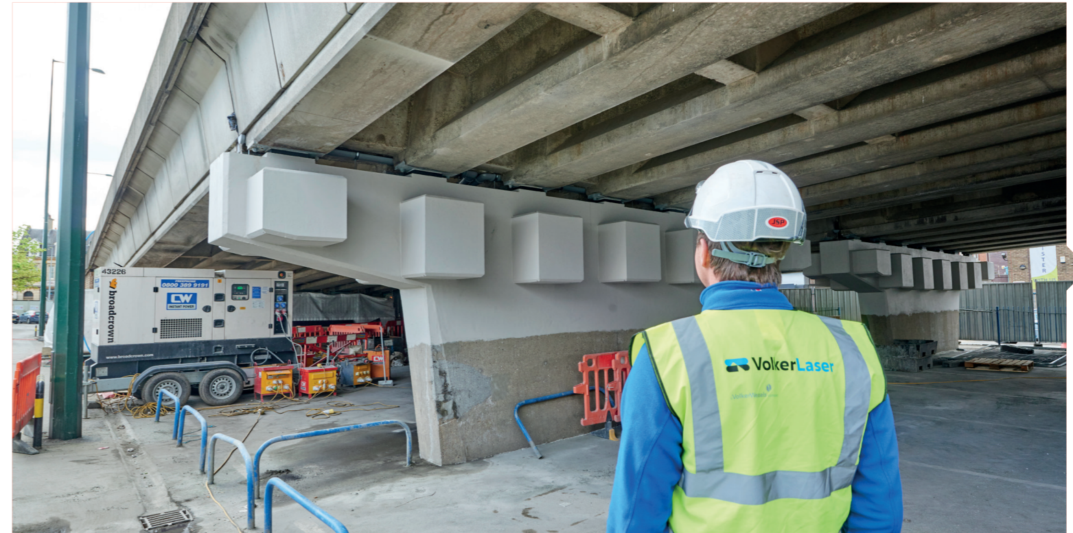
THE CLEETHORPES ROAD OVERBRIDGE AFTER BEING STRENGTHENED AND REFURBISHED
