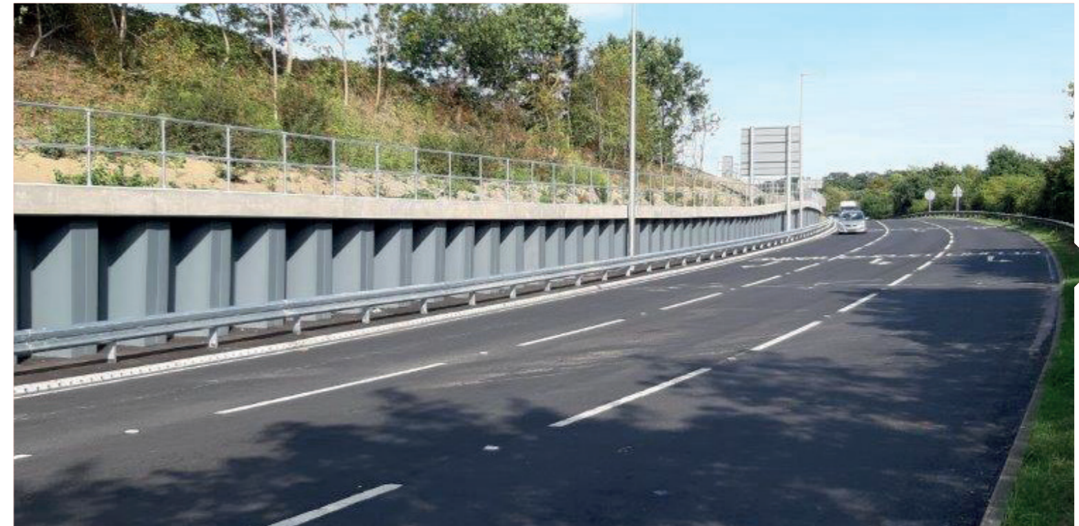
A3 STOKE INTERCHANGE SLIP ROAD WIDENING AND HIGHWAY WORKS
